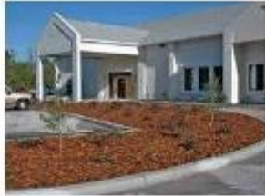
Fellowship Center Entrance
