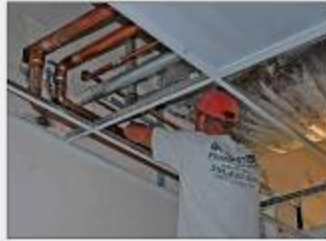
Plumbers are making final connections and testing all water lines.
