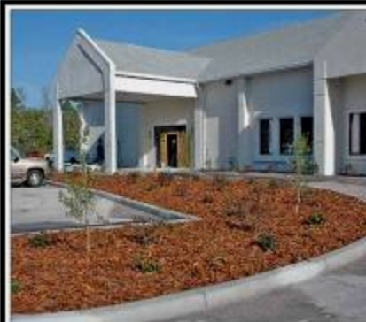
Landscaping has been completed adjacent to the new fellowship center, and around the perimeter of the property in the area of the new Fellowship Center.
