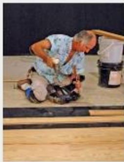
Southern yellow pine flooring installation is underway in Fellowship Hall.
