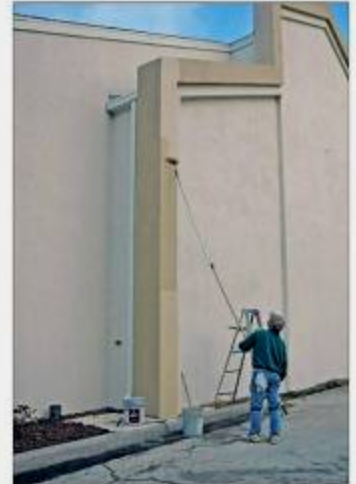
Outside painting is nearing completion, and contrasting trim color is being applied to highlight the architectural features of the Fellowship Center structure.
