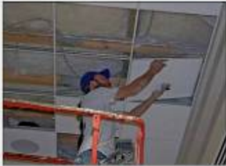
Acoustic ceiling tile being placed in Fellowship Hall.
