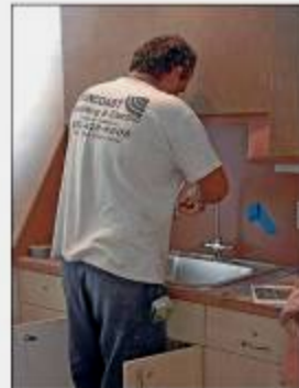
Faucets are being installed on the sink at the beverage counter in the entrance to Fellowship Hall.
