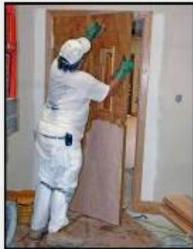
Workers apply stain to wood doors and casings in the new Fellowship Center.
