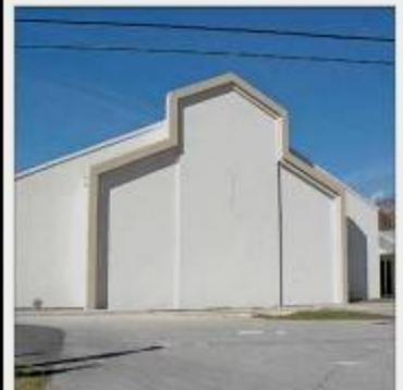
The end result is apparent. A new flame and cross emblem will soon be added to the end wall to complete the outside appearance.
