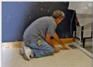
Vinyl floor tile being laid in several rooms adjacent to the stage and Fellowship Hall.
