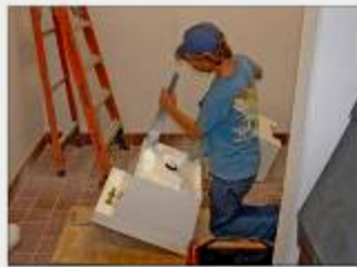
A utility sink is being assembled for installation in the dishwashing area of the new kitchen.
