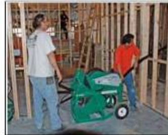
Once the rope is in place, heavy gauge wire will be attached and pulled and pushed through the conduit using special machinery. (Left) Shown inside.
