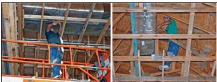
Installed duct work is being insulated in the ceiling.
