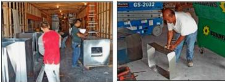
Large Air Conditioning and Heating ducts are being prepared for installation in the Fellowship Hall Ceiling.
