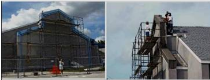
Architectural elements are being added at the front of the new Fellowship Center. This front area will include a new lighted UMC Flame and Cross symbol.
