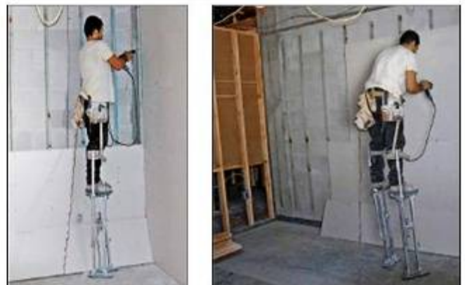
Stilts make it easier to reach the top of the panels. Now the finished room size and shape of the interior is readily apparent with the addition of the sheetrock.
