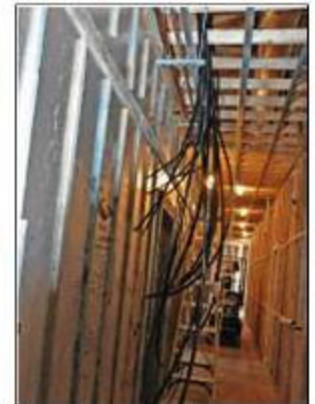
(Right) Just a few of the many large cables pulled into the building now hang in the corridor waiting to be attached to power supply boxes.
