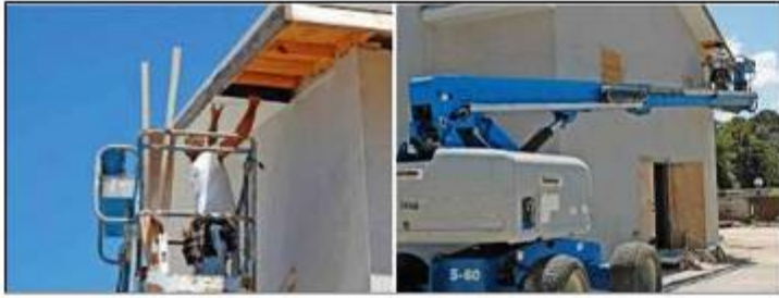
Soffits being installed at the junction of the roof and wall throughout the new buildings.
