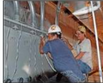
Unbelievably large amounts of wire are required to supply electricity to the new Fellowship Center. (Left) Electricians are pulling string, then rope through the conduit.
