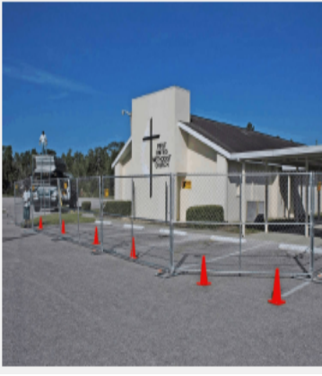
Construction fencing is being erected to protect the construction site and maintain safety.
