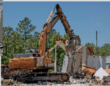
The sequence of seven photos above document removal of the entrance - the final piece of the old structure to be demolished. The roof is peeled off with a single swipe of the grapple, then the wall is pushed over, and finally, the steel posts that supported the roof are lifted down.
