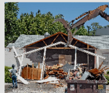
The sequence of seven photos above document removal of the entrance - the final piece of the old structure to be demolished. The roof is peeled off with a single swipe of the grapple, then the wall is pushed over, and finally, the steel posts that supported the roof are lifted down.
