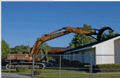
Shortly after 7:30 AM the excavator operator lifted his grapple up over the fellowship hall roof, plunged it down through the roof, then pulled it out through the side wall - and the demolition process was underway (three photos above and right).
