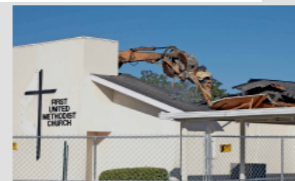
The roof was systematically shattered, the debris lifted out and placed in a container. When the roof debris was cleared, the surrounding walls were knocked down and the concrete debris piled for recycling.
