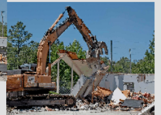
The sequence of seven photos above document removal of the entrance - the final piece of the old structure to be demolished. The roof is peeled off with a single swipe of the grapple, then the wall is pushed over, and finally, the steel posts that supported the roof are lifted down.
