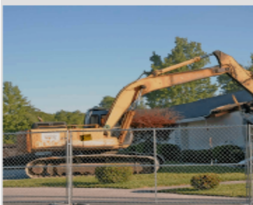
Shortly after 7:30 AM the excavator operator lifted his grapple up over the fellowship hall roof, plunged it down through the roof, then pulled it out through the side wall - and the demolition process was underway (three photos above and right).
