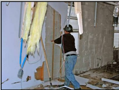
Don of SDC removing sheet rock from walls.
