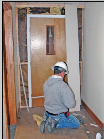
Left: A temporary wall across the width of the old building was erected to separate the fellowship hall/kitchen/vestibule area - which will be completely demolished - from the former restroom/library/thrift shop work room area - which will be extensively renovated. The wall is visible from the Administrative wing.
