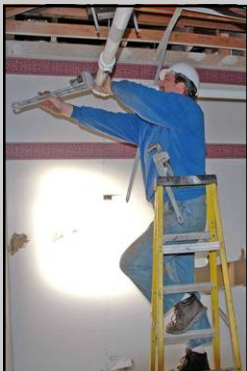
Brian, of Frontline Fire Protection Inc. removing fire sprinkler pipe in former restrooms.
