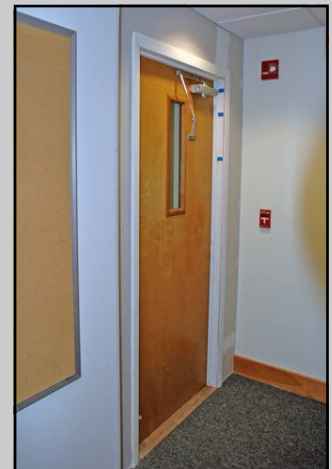
Left: Jim installing a new door to separate the construction area from the Administrative Building .
