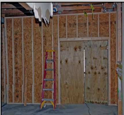
Left: A temporary wall across the width of the old building was erected to separate the fellowship hall/kitchen/vestibule area - which will be completely demolished - from the former restroom/library/thrift shop work room area - which will be extensively renovated. The wall is visible from the Administrative wing.
