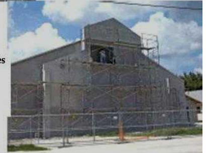
Right: ...but the final coat provides a smooth and even finish for the paint that will then be applied.
