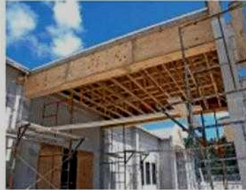
Below: The ceiling being framed-in under the drive-through roof, and electric conduit is being installed for lights.
