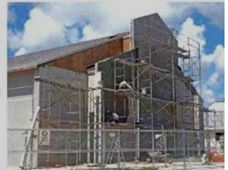
Right: From scaffolding, workers apply stucco on the Bradshaw Street side.
