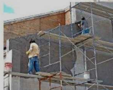
Left: The first coat is heavy...
