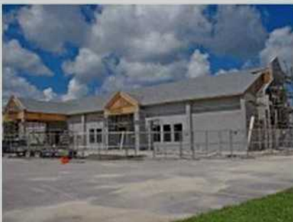
Left: And the new Fellowship Center has been "dried in", as the contractors say.
