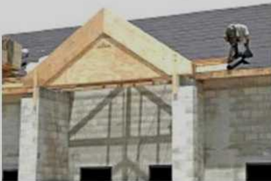
Left: Roofing paper goes on as the first step in the process of completing the roof.
