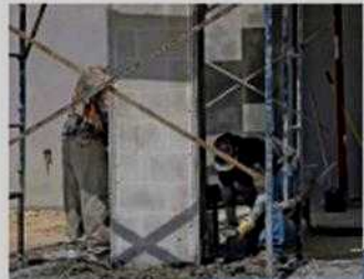
Above: Workers begin to apply stucco to the roof pillars.
