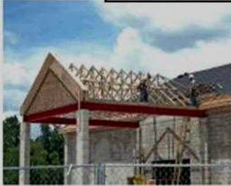
Left: Roof trusses are installed for the entrance roof.
