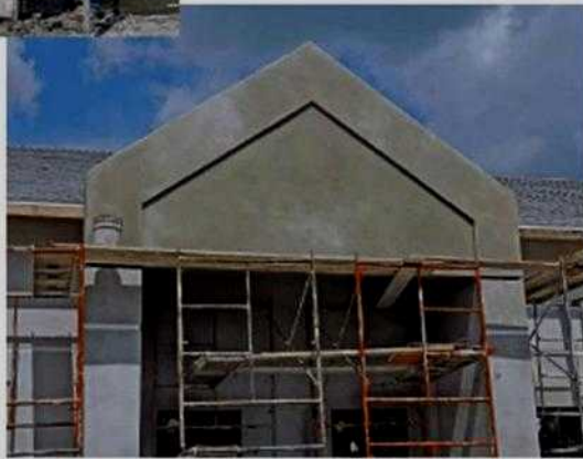
Above: Workers begin to apply stucco to the roof pillars.
