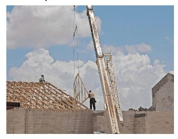
A main roof truss for the fellowship center is swung into place, then fastened securely by workers high up in the roofing. Roof truss installation began on July 17 and was essentially complete (including plywood sheathing) by July 25.
