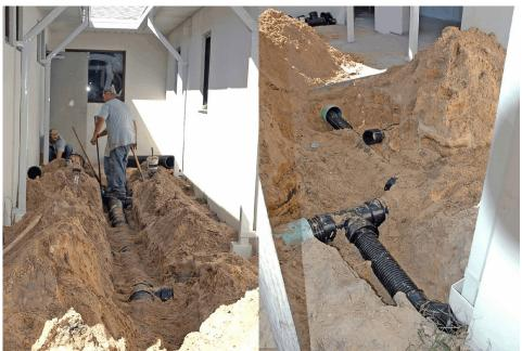
Rain water from the roofs of both the new Youth Center and the Administrative Building funnel into the narrow space between these two buildings. The volume of water there could be very high during heavy rains, so all of the down spouts are being connected to a large drain pipe that will move the water away from the buildings and avoid problems of the water seeping inside. The three photos above show the ditch for the drain pipe, and the various down spout connections to it.
