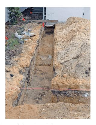
Batter Boards and string used to lay out the location and elevation of the concrete foundation (two photos above).
