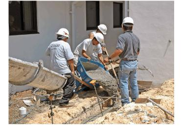
The concrete is leveled after pouring to support the block walls that will be added later.
