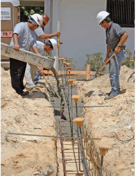
Trenches with rebar are poured w i t h concrete to form the building foundation.
