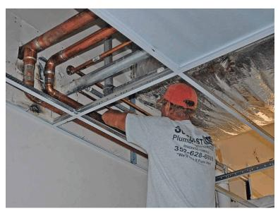
Plumbers are making final connections and testing all water lines (photo at left).
