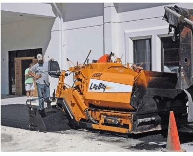
dumped into the paving machine, and laid down in the driveway approach to fellowship hall.
