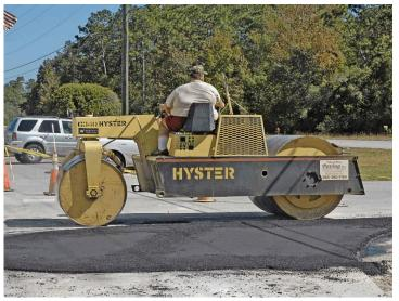
At the Bradshaw entrance to the west parking lot, asphalt is laid down by the paving machine, edges touched up by several workers, and then rolled to compress it to the same level as the surrounding pavement.
