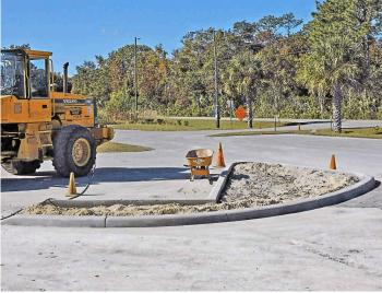
Lime rock that was the foundation for the former blacktop is being removed to make way for topsoil (above left). A small bed that will be planted with shrubs has been neatly outlined by the concrete curbing (above right).
