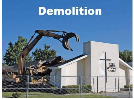
Demolition of the front wall of the old fellowship hall, including the First United Methodist Church lettering, occurred early in the morning of April 17. That wall was quickly reduced to rubble, as the excavator operator simply swung the mammoth grapple against the wall and pushed it over. It was an unsettling moment, relieved only by the knowledge that a new, larger, state-of-the-art fellowship center would soon rise in its place.
