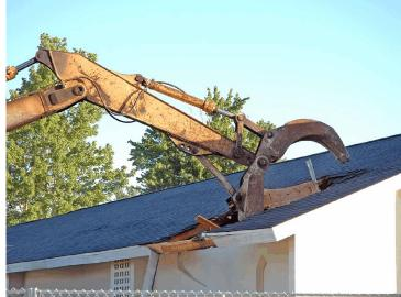
Shortly after 7:30 AM, the excavator operator lifted his grapple up over the fellowship hall roof, plunged it down through the roof, then pulled it out through the side wall - and the demolition process was underway (three photos above and right).
