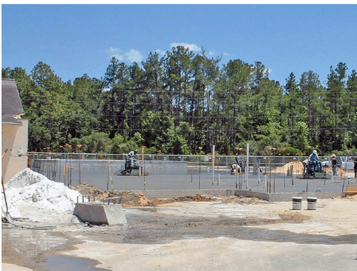
Fellowship hall floor finishing (below left) and block wall and door frame installation (right)
