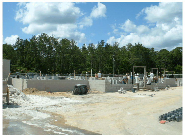
Fellowship hall floor finishing (below left) and block wall and door frame installation (right)
