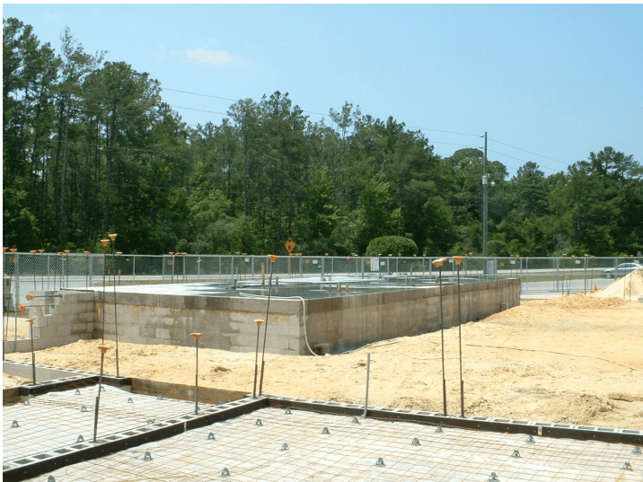
Fellowship hall floor finishing (below left) and block wall and door frame installation (right)
