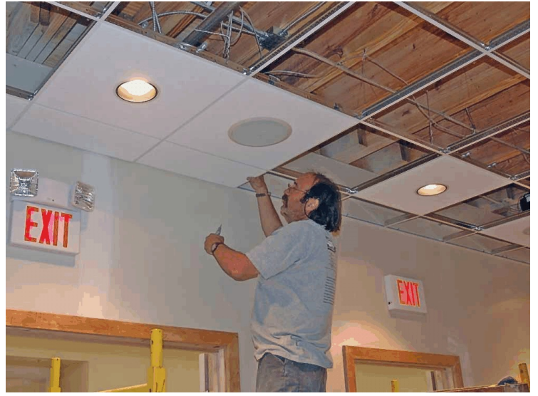
Acoustic ceiling tile being placed in fellowship hall (two photos above).
