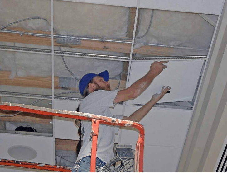
Acoustic ceiling tile being placed in fellowship hall (two photos above).
