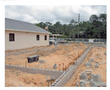
Concrete blocks are being laid on the poured concrete foundation, and the outline of the new rooms quickly becomes apparent. Shown here: the youth room walls (above right); stage walls (raising the stage above the level of the rest of Fellowship Hall - two photos below); Thrift Shop (bottom left); Mechanical Room (bottom right).
