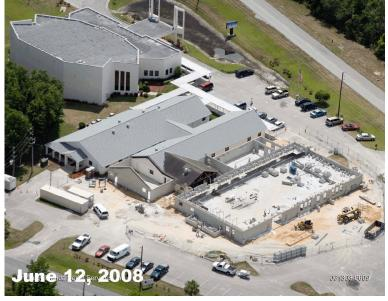
June 12, 2008 (photo at left). Slabs for the floors of all rooms have been poured, and concrete block walls are being erected. Walls for the new thrift shop are complete, included the gable end. The other walls are nearing 10 feet in height, which will be their finish height except for the fellowship hall, which will be 16 feet high.
