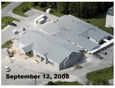
September 2008 (photo at left). Stucco has been applied on the exterior walls, and the roof is essentially complete. From this point on, there will be little further change to the exterior of the building until paving and landscaping occurs. But much work is underway inside.
