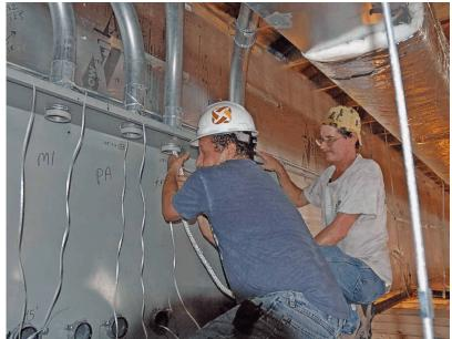
Unbelievably large amounts of wire are required to supply electricity to the new Fellowship Center. In the photo at left, electricians are pulling string, then rope through the conduit.
