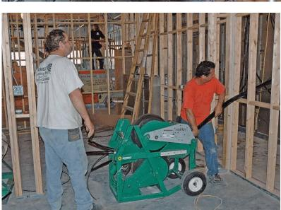
wire will be attached and pulled and pushed through the conduit using specialized machinery, shown inside (middle photo), and outside (photo at lower left).
