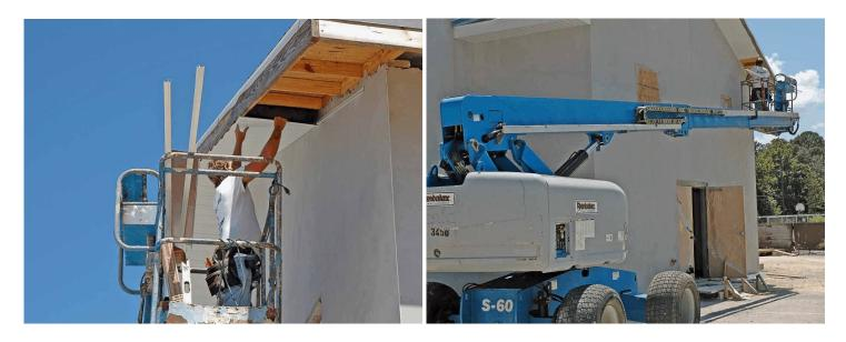
Soffits being installed at the junction of the roof and wall throughout the new buildings (above).
